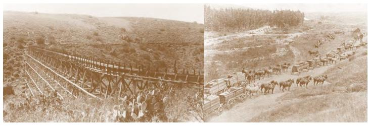
In 1885, the sole source of water in the area was from wells with windmills. By 1886, the Cuyamaca earthen dam was built and construction of the flume began. This monumental endeavor used nearly nine million board feet of redwood lumber, which required 100 wagons, pulled by 800 mules and horses, for its transportation from San Diego harbor inland.
